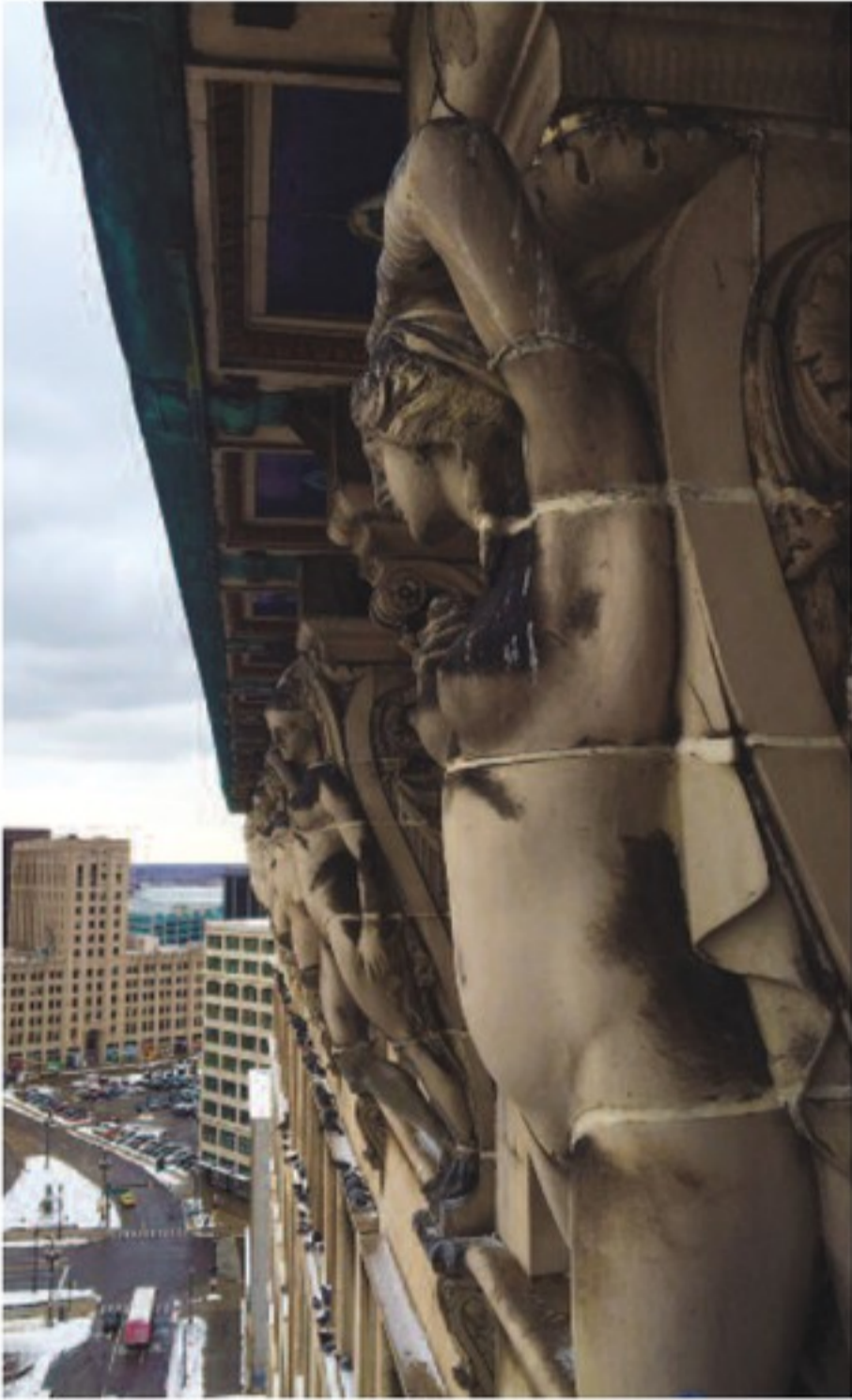
Left/Middle: Removed in 2016, the damaged terra-cotta sculptures had been architecturally supporting the cornice of the Book Building, circa 1917, for just under a hundred years. Each of the 13-foot-tall female sculptures, called caryatids, is now replicated in fiberglass.
